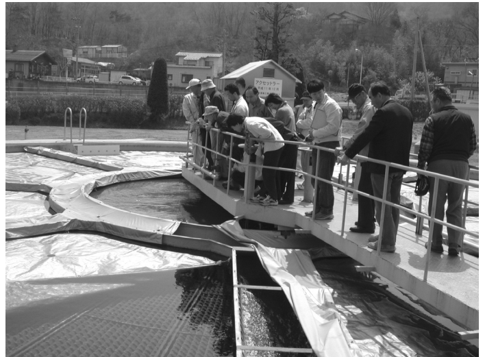
県営水道諏訪形浄水場
